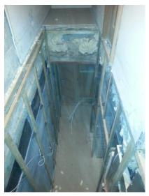
With a new concrete floor, the basement was waterproofed using a cavity drainage membrane system, linked to a sump with two pumps and a high
