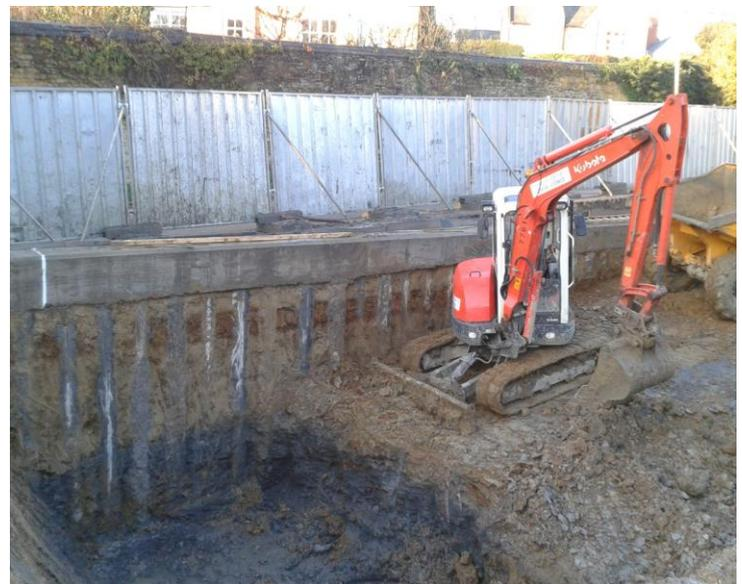
Once the piles were finished beautiful basements moved in to finish off the site stabilisation by installing the pile capping beam.
